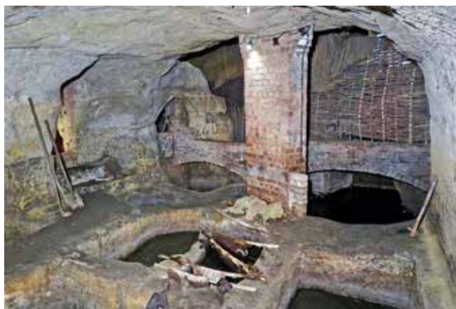
Broadmarsh Caves: Tannery pits cut into the sandstone floor. Photo Clive Penfold
